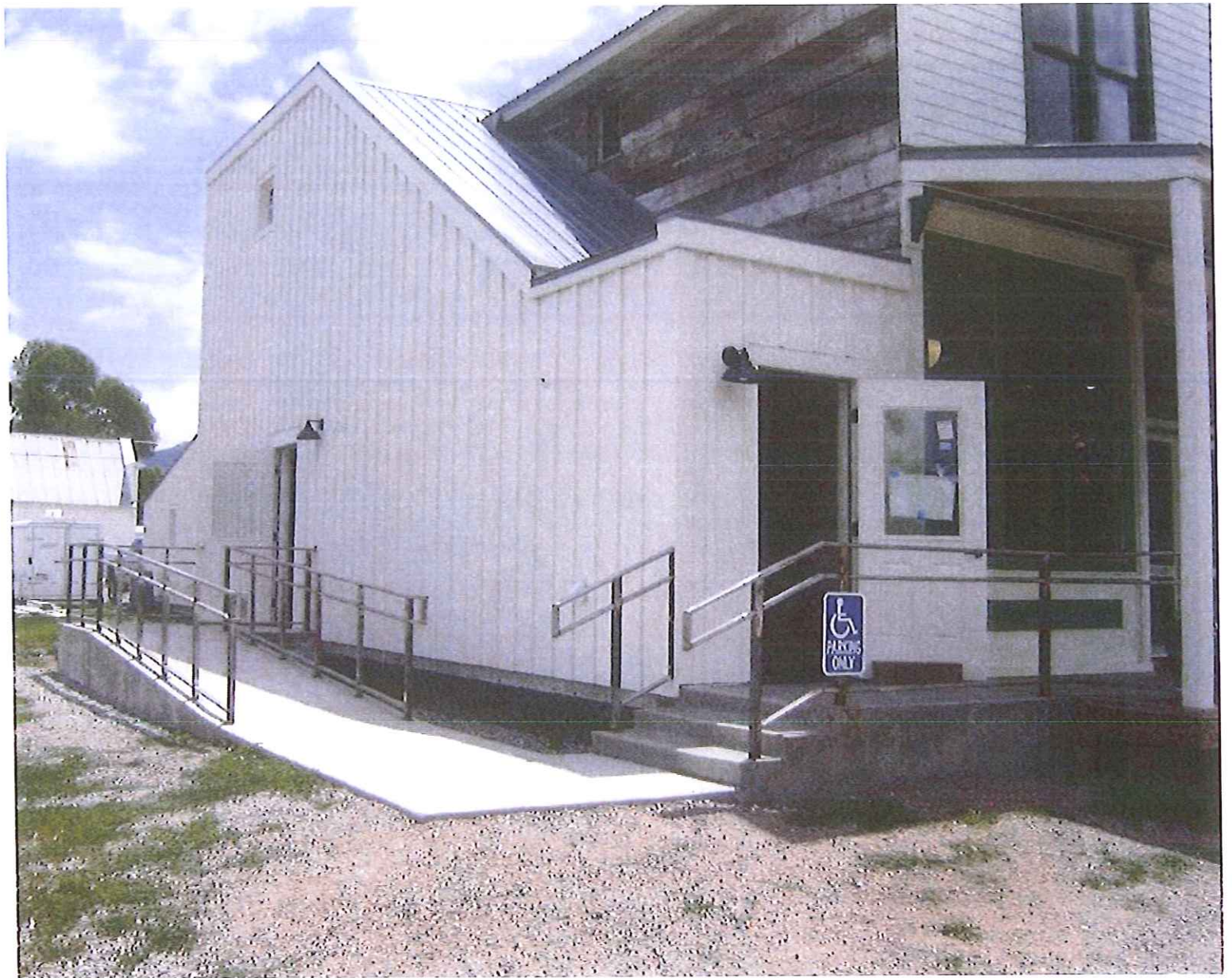
Crossan's elevator location in relationship to stairwell entrance entrance.
