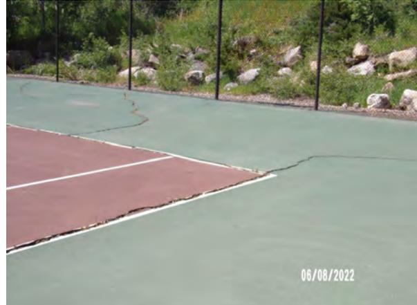
Below: Cracks from removed netting poles (Left)
