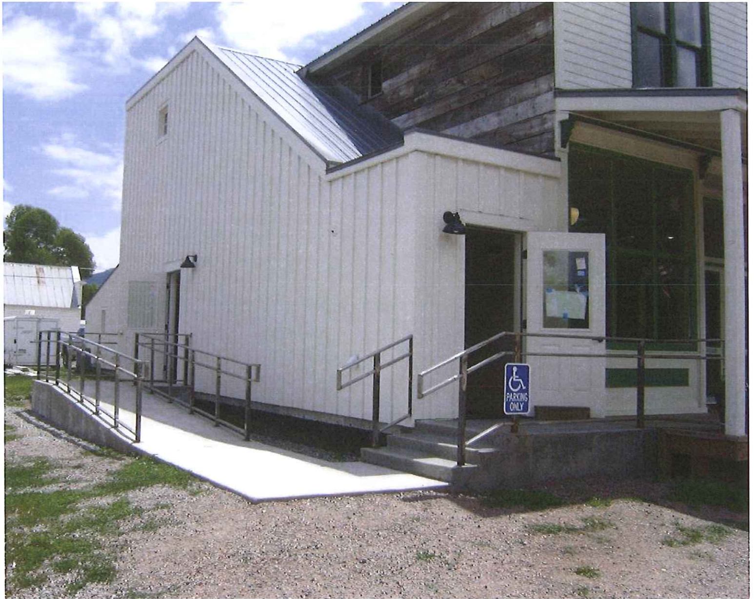
Crossan's elevator location in relationship to stairwell and entrance.
