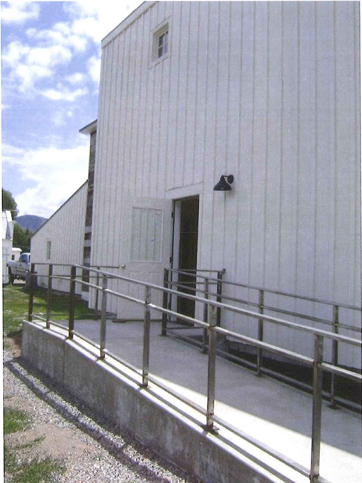
Crossan's - elevator location
