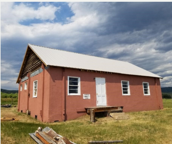
Elkhead Community Center South Facing Side, June, 2021
