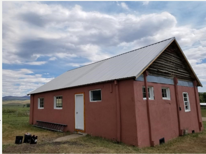
Elkhead Community Center North Facing Side, June 2021
