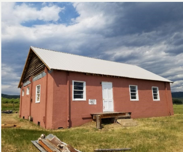
Elkhead Community Center South Facing Side, June, 2021
