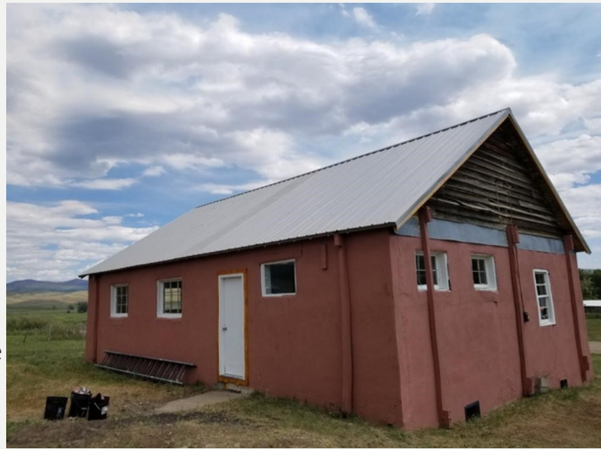
Elkhead Community Center North Facing Side, June 2021
